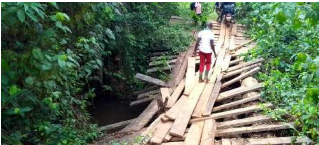
Figure 6: Bridge on the main road linking the target zone to the interior of the country, 27 February 2024, IDCocoa
